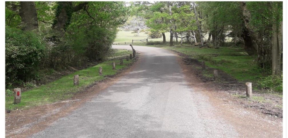
Verge restoration, before and after.
