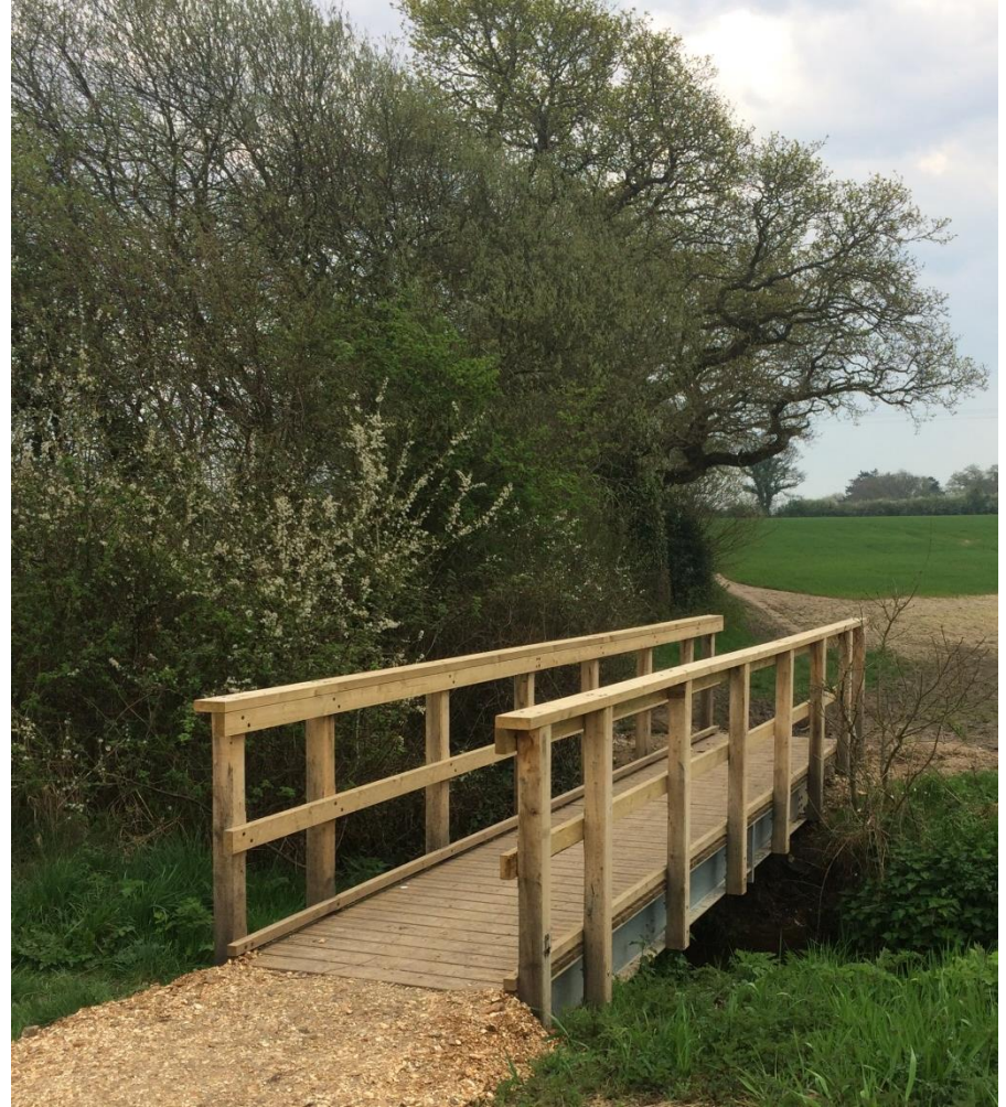
LYMINGTON & PENNINGTON FOOTPATH 59 & BRIDGE
