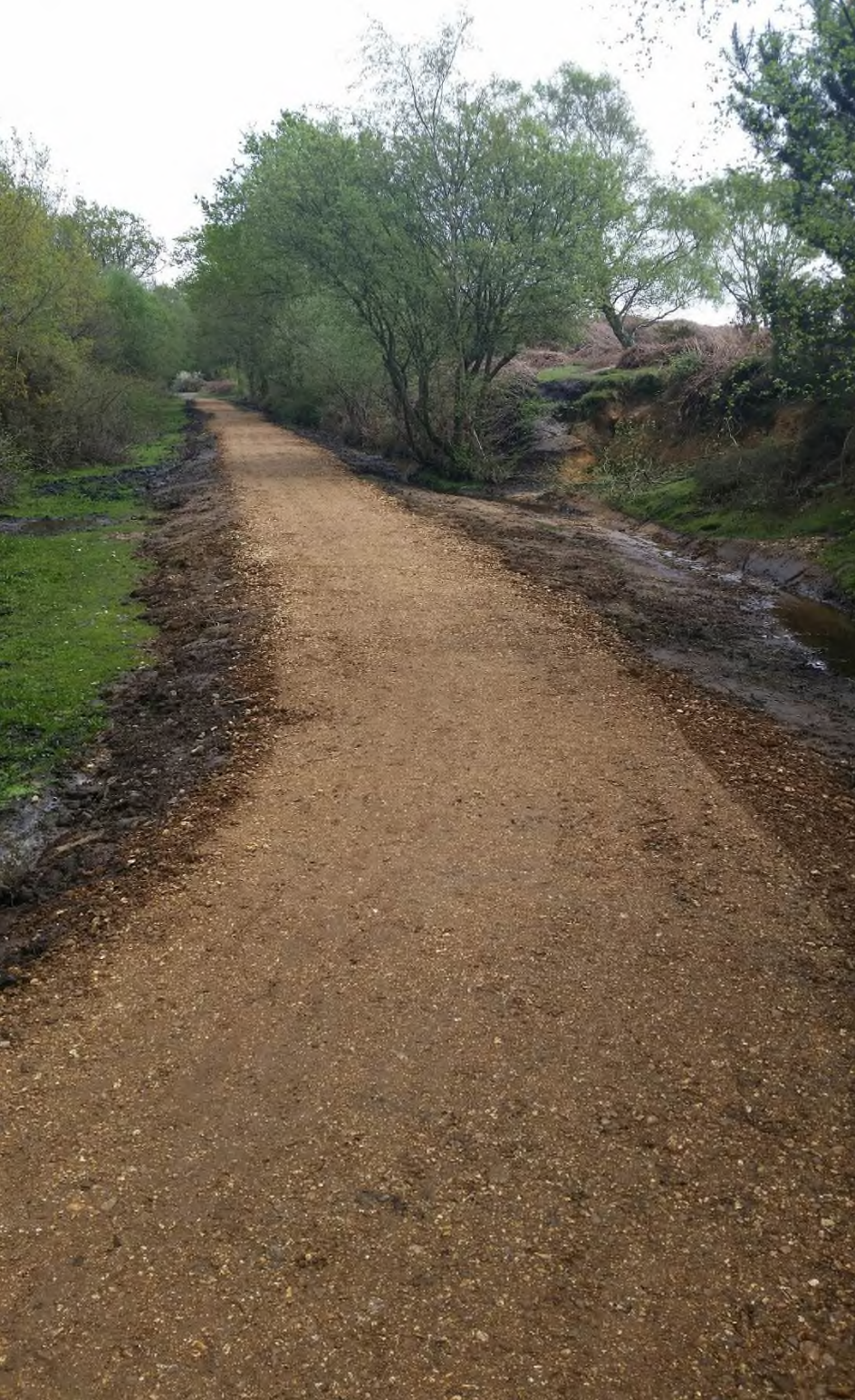
Finished raised track with softened edges.
